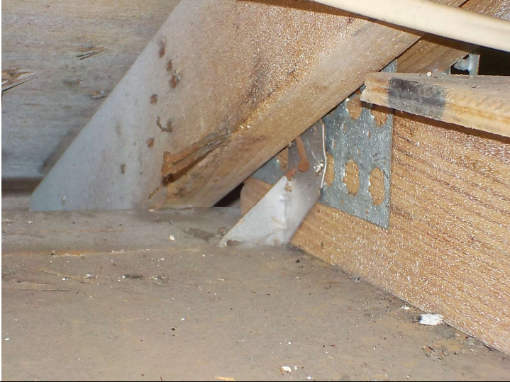
Roof To Wall Connection
