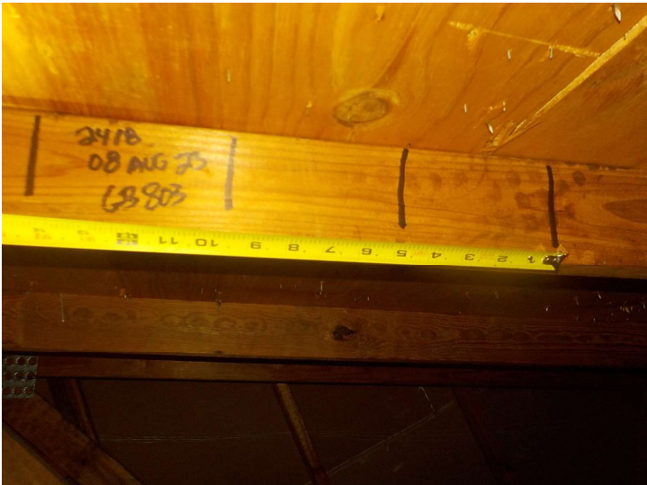
Roof Deck Fastener Spacing
