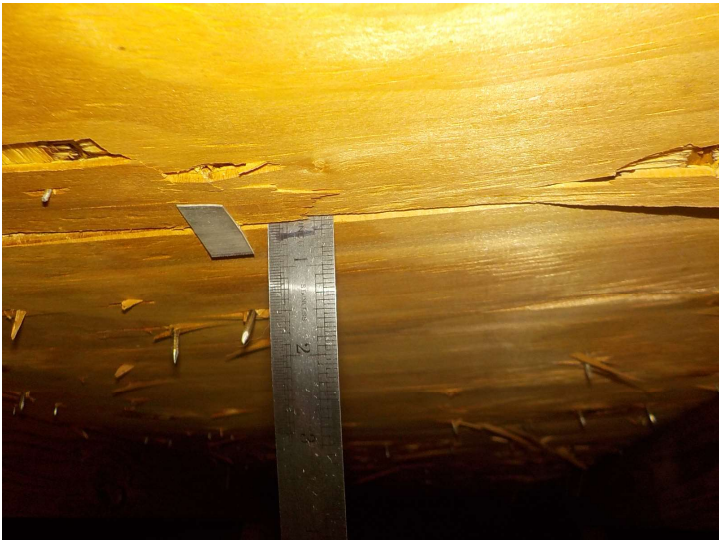
Roof Deck Thickness 1/2 inch plywood
